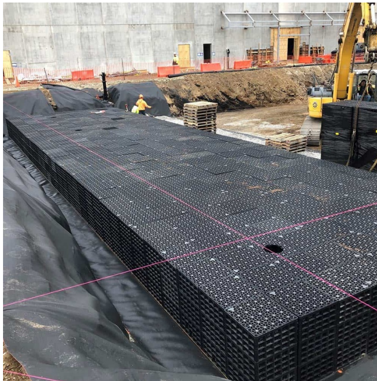
Figure 2: R-Tank being installed at a site for stormwater storage.
