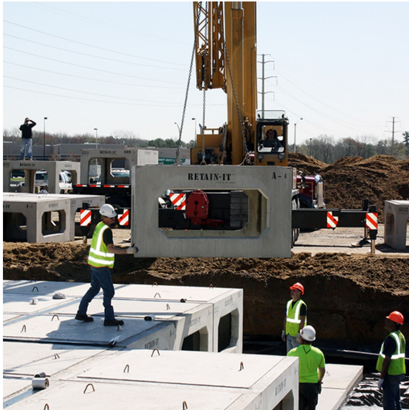
Figure 3: Retain-It stormwater detention basin being installed.
